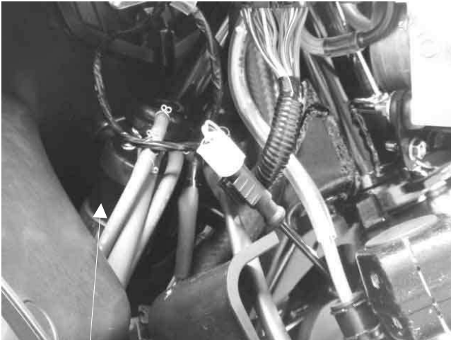
Charcoal Canister/ Purge Control Valve
