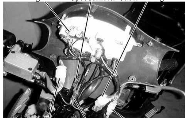
Lighting/ Start Wires
